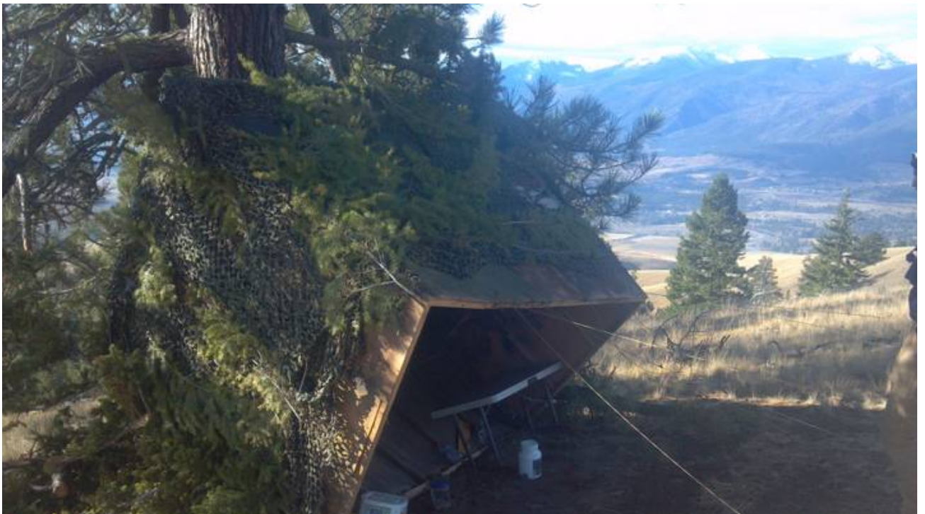
During a period of particularly high winds, our blind was lifted off its foundation. Were it not for the large pine just behind, it's likely our blind would have been blown down into the draw to the south.
